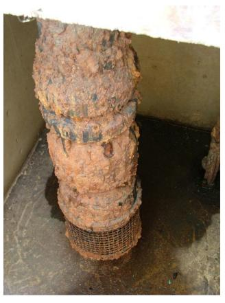
Figure 2: Old Cooling Tower Pipe
