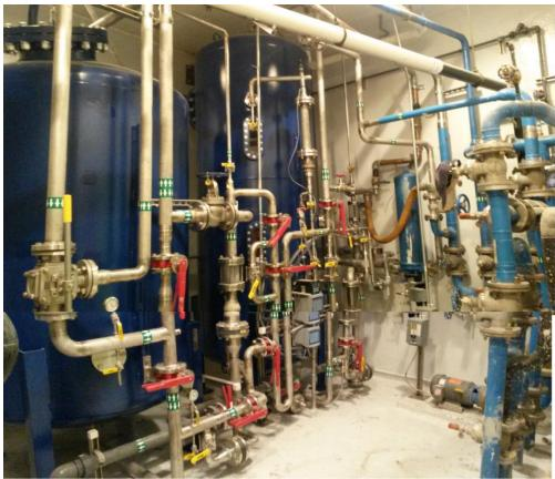
Figure 7: New Demineralizer System
