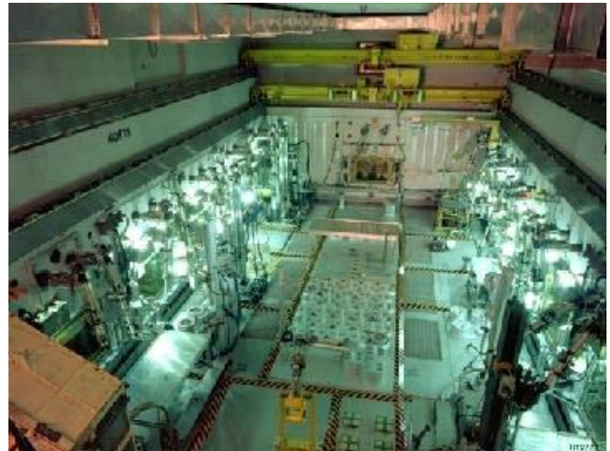
Post Irradiation Examination (PIE) Facilities at Materials & Fuels Complex (MFC @ INL)
