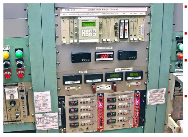
Each channel provides short reactor period scram & high reactor power scram Each channel utilizes one fission chamber for widerange power operation Reactor power and period calibration and scram checks can be done with the reactor operating Test signal travels along the detector signal path starting from the fission chamber pre-amplifier
