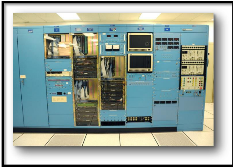
Reactor Control System
