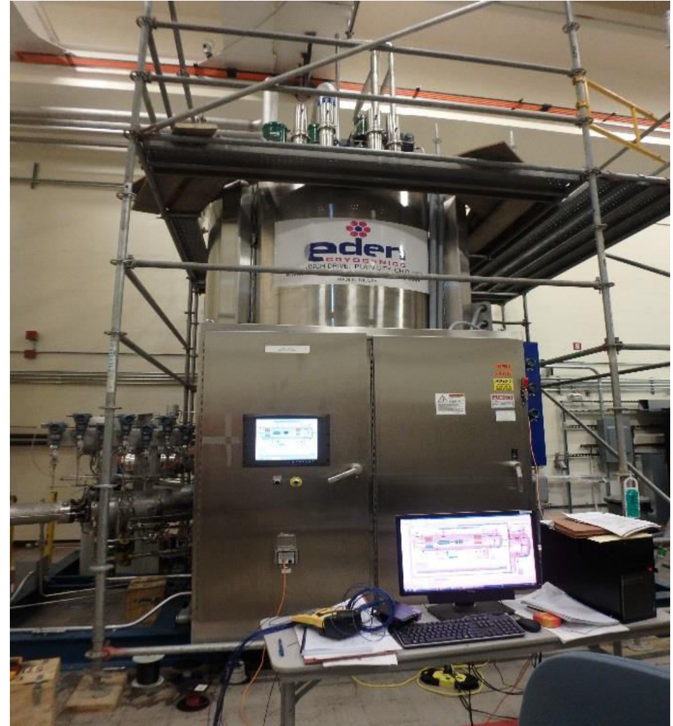
Attached PLC Panel to Coldbox Enclosure, continued field wiring and PLC programming.
