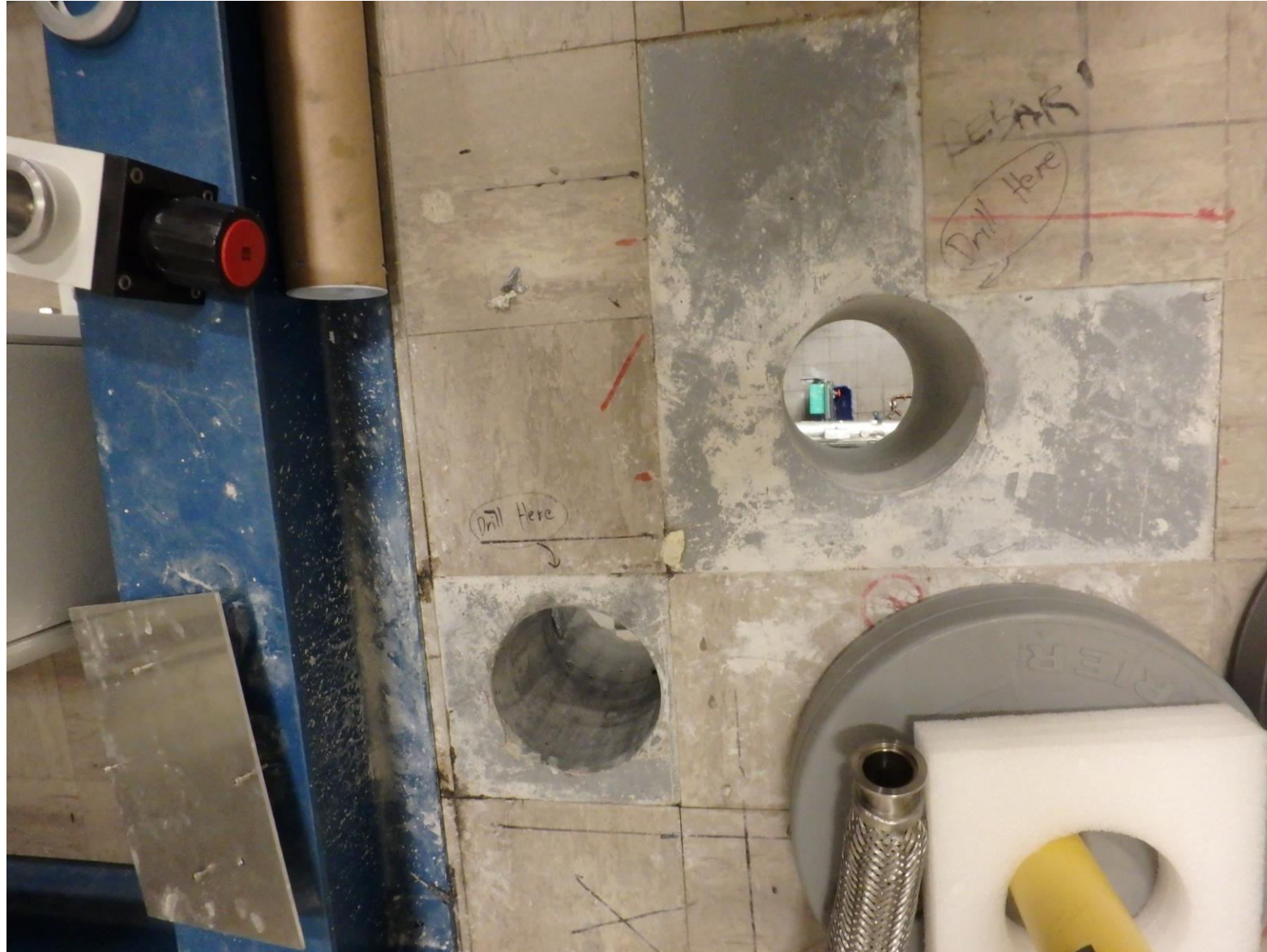
Drilled holes in Floor for Helium Load Lines, Dec/2016.
