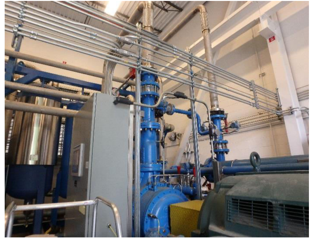
Plumbing and Wiring Completed and Successful Start of Compressors, Sep/2016. Required resetting the Soft Starter and Adjusting of Network Protective Switch.
