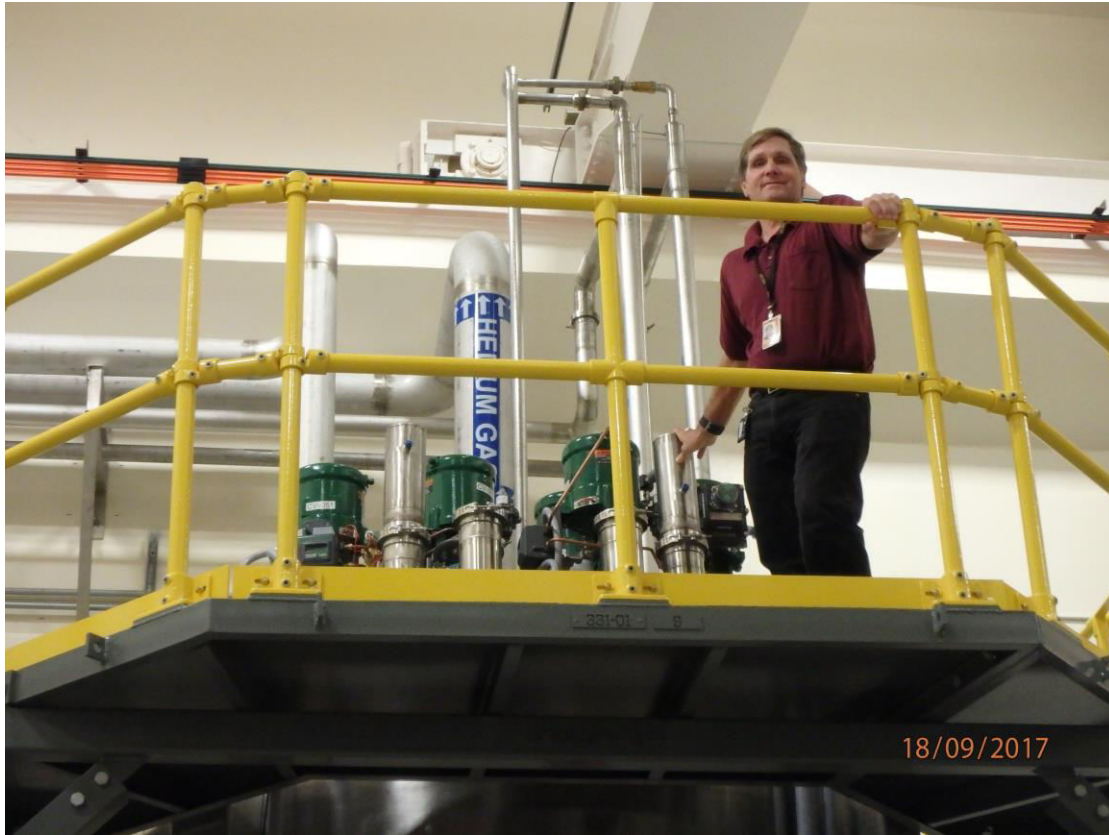
Catwalk Installed around Coldbox, Aug/2017.
