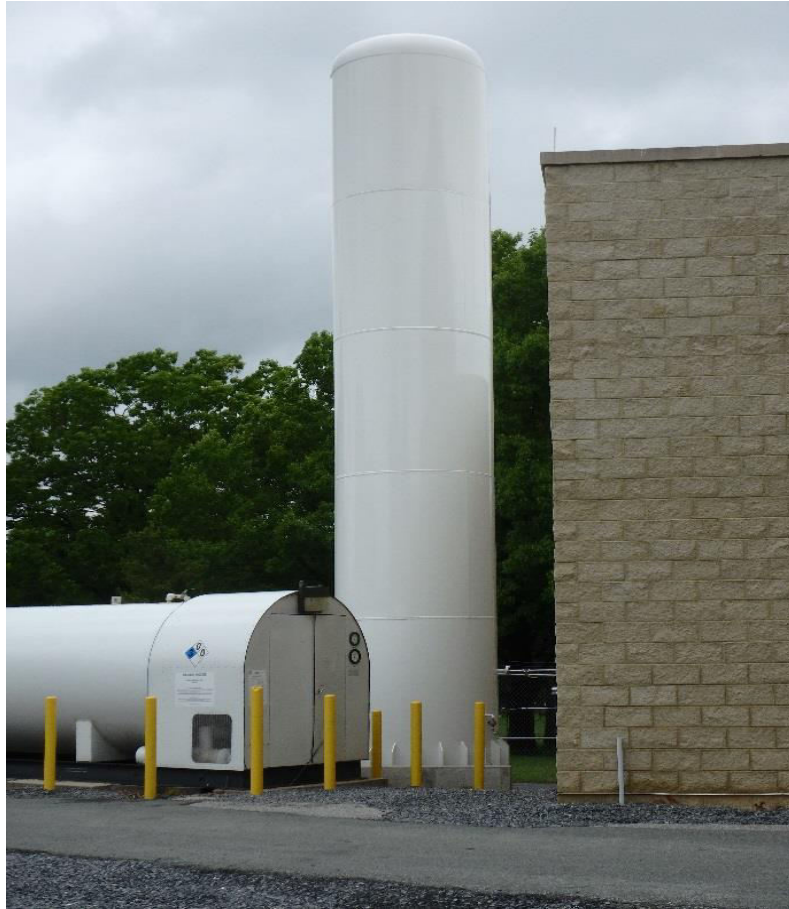
Helium Reserve Tank, Connection to Oil Removal Skid and Connection to High Pressure Makeup Tanks, Received Nov/2015.
