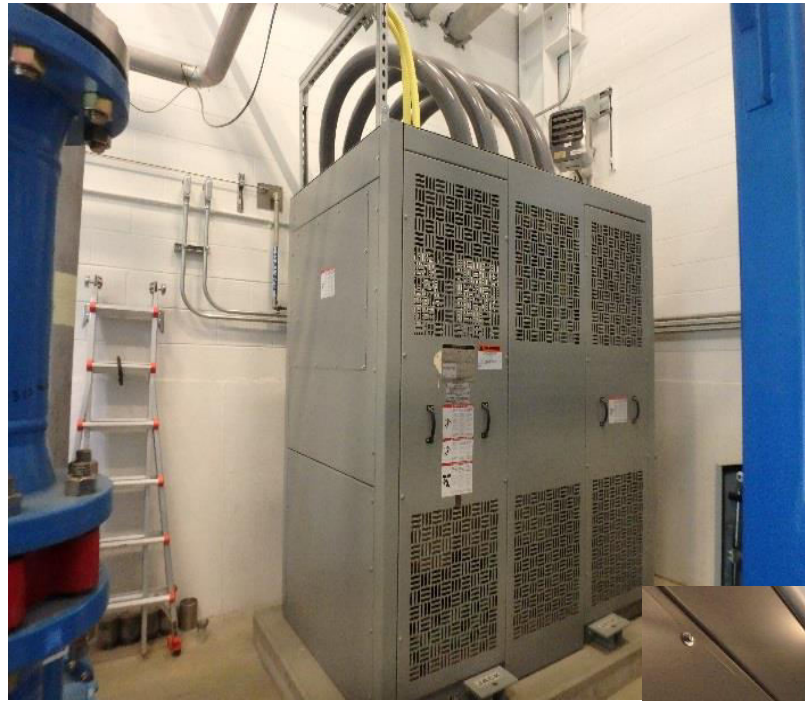
480V/4160V Step-up Transformer and Power Cables received Feb/2014
