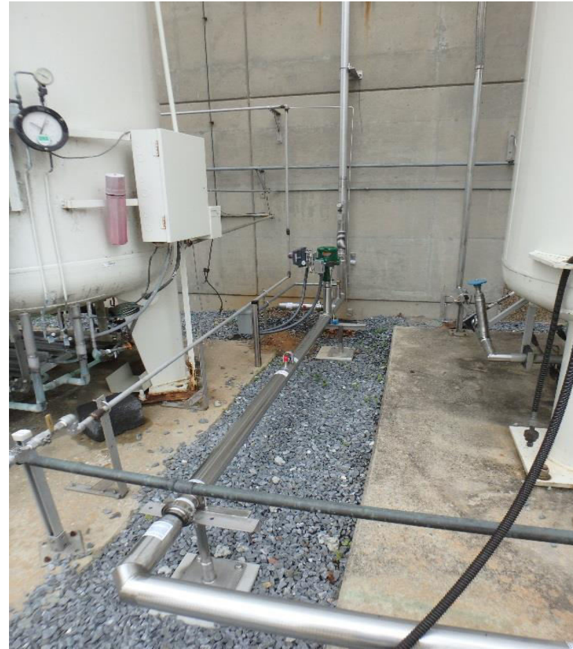
Connection Piping for LN2 Tank and Emergency Shutoff Valve, Installed Aug/2016.
