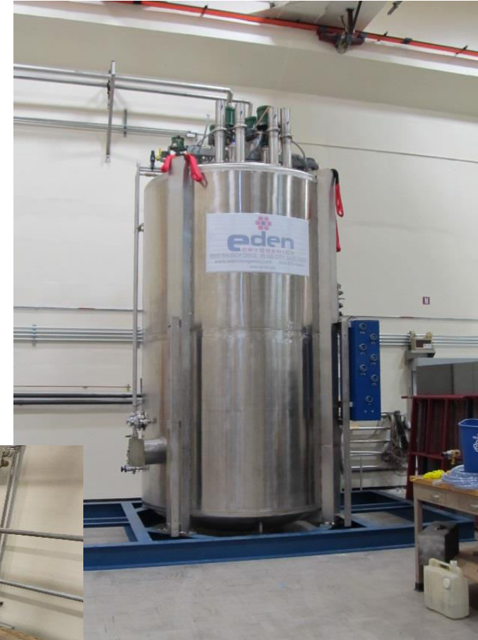
Support Frame made, Coldbox Attached in place in C200.
