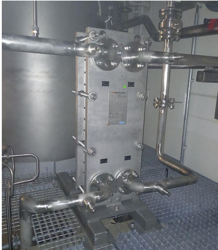
Figure 3: Heat exchanger of the 99-Mo system, mounted in front of the primary/secondary heat exchanger in the so called primary cell of FRM II.
