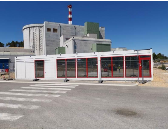
Figure 1a: JHR support building. v2019, July
