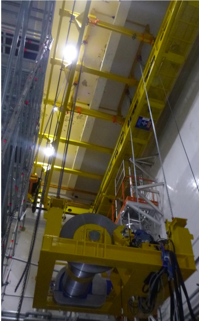
Figure 4: hoisting of the new hoist in 2022
