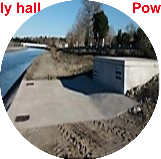
3rd cooling system
