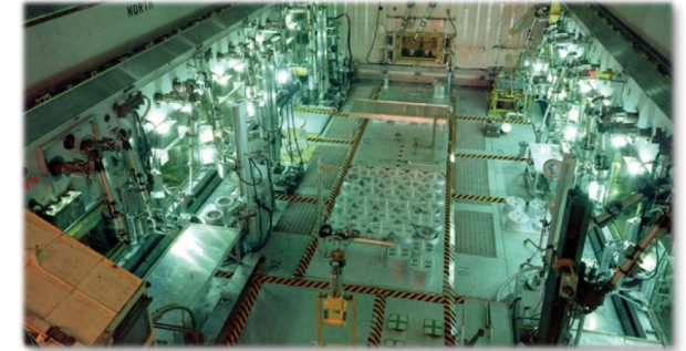
Hot Fuel Exam Facility
