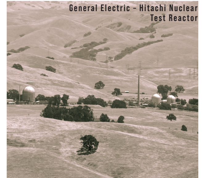
General Electric - Hitachi Nuclear Test Reactor April 18 - 20, 2023. The inspection included a review of procedures, experiments, health physics, design changes, committees, audits and reviews, maintenance logs and records, and transportation. No violations were identified. ML23159A013
