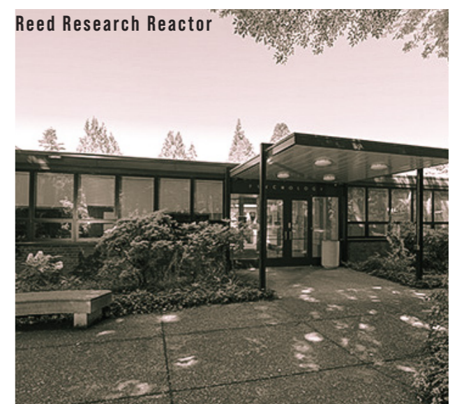
Reed Research Reactor April 17-20, 2023. The inspection included a review of organization and staffing, operations logs and records, requalification training, surveillance and limiting conditions for operation, experiments, emergency planning, maintenance logs and records, and fuel handling logs and records. No violations were identified. ML23186A133
