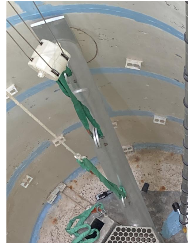
Evaluation of fit of inner section of beam port
