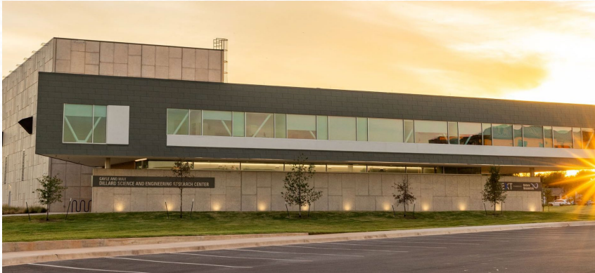
Completed MSR-1 facility at Abilene Christian University (ACU)
