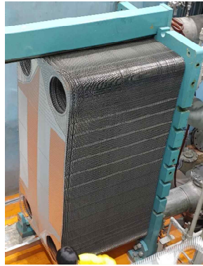
(a) HANARO Heat Exchanger
