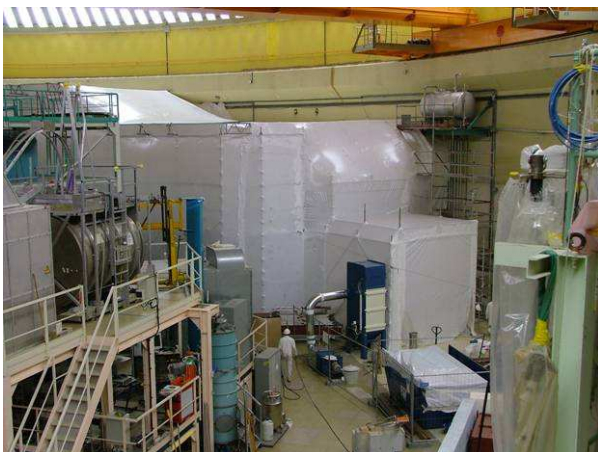
Figures 8 and 9 - Containment of structures during phase 2 of dismantling operations
