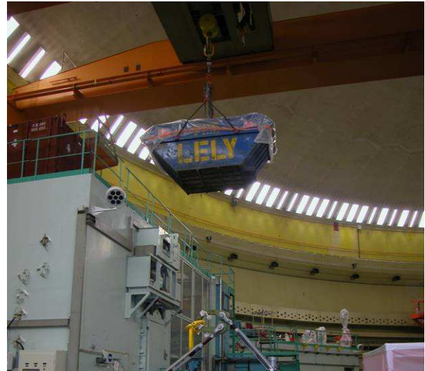
Figure 12 – Removal of a skip of debris using the overhead crane
