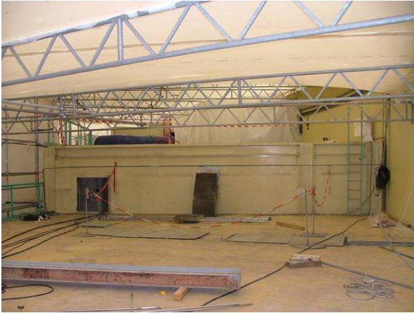
Figure 11 – Containment of roofs of buildings during phase 2 of dismantling operations
