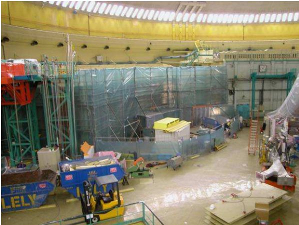
Figure 7 – Containment of structures during phase 1 of dismantling operations
