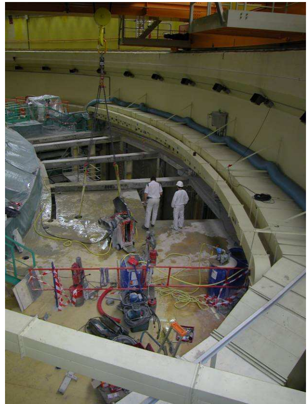
Figure 6 – Wet sawing of roofs of buildings
