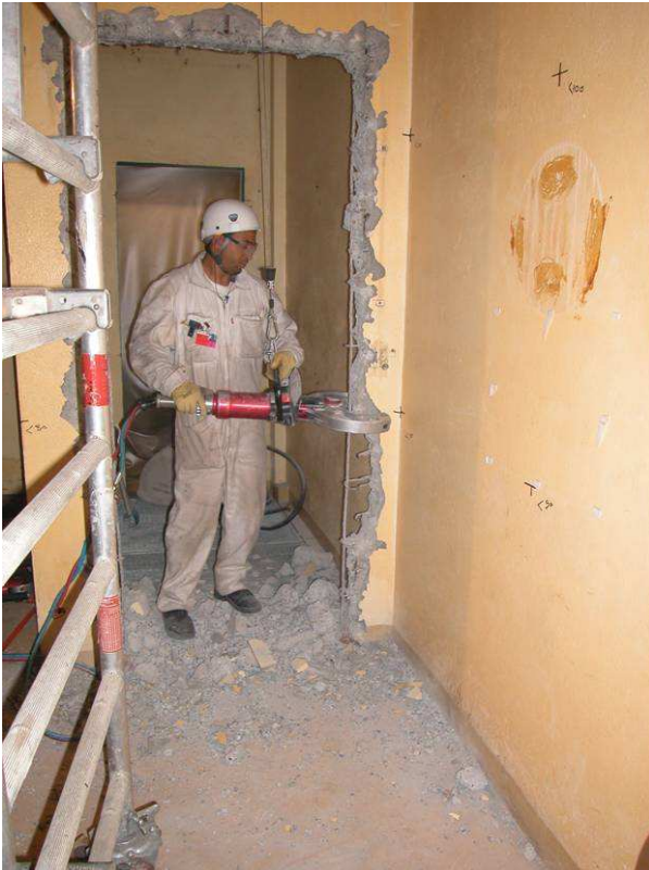
Figure 5 – Hydraulic nibbling of walls
