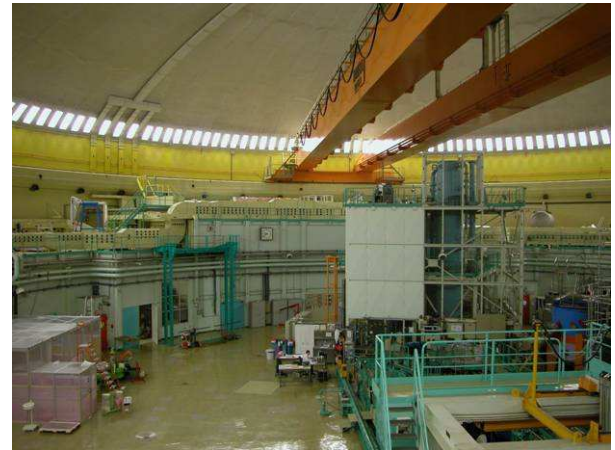
Figure 3 – View of part of the masonry structures around the edge of the reactor building
